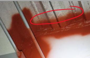
The UL assembly is tested with bare metal. By applying the spray fire stopping onto the overspray, the adhesion is likely compromised by the spray fireproofing.
